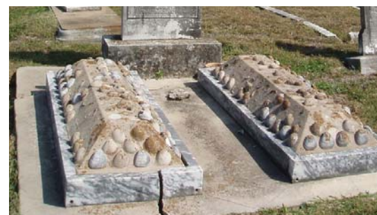
Figure A-38. These shell-encrusted plot covers suffer from cracking due to subsidence and also loss of most of their shell ornamentation (NB). JMA, 2009.
