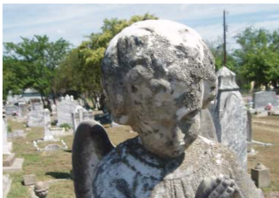
Figure 4-42. Lichen, although slow-growing, can damage soft materials, such as this marble. JMA, 2009.
