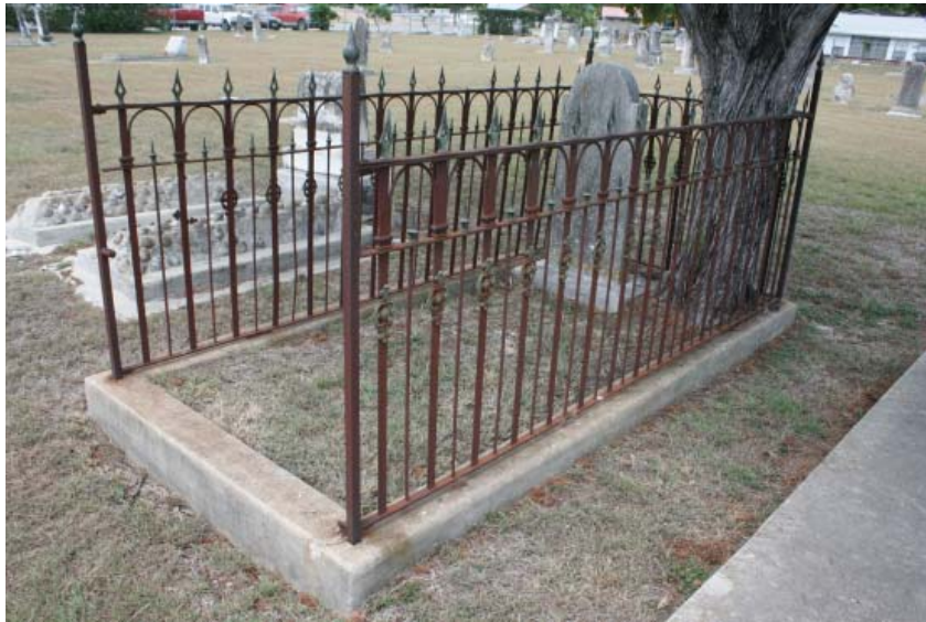
Figure 4-54. The gate has been removed from this plot fence. JMA, 2009.
