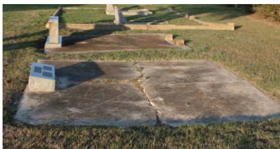
Figure A-18. Two family plots that have been covered by poured concrete (NB). Note that the shrink-swell tendency of the soil has led to cracking. JMA, 2009.
