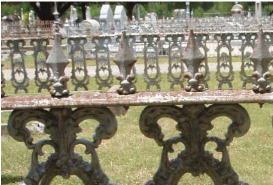
Figure 4-52. Cast iron fence that has been painted silver. JMA, 2009.
