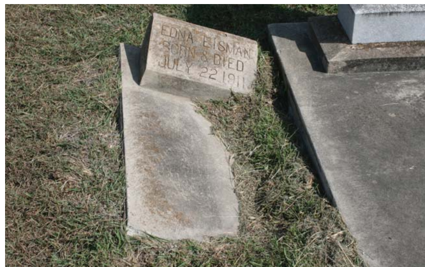
Figure 1-9. The subsidence of this grave cover and headstone in the New Braunfels Cemetery is the effect of their placement within Houston Black clay. JMA, 2009.
