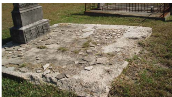
Figure A-21. This concrete topping failed due to issues of ponding where water pools and seeps into masonry (NB). JMA, 2009.
