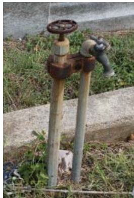
Figure 5-62. This fixture may indicate the location of a valve. JMA, 2009.
