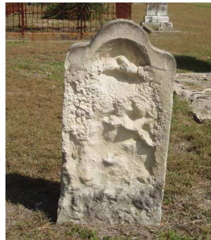
Figure 4-39. Severe erosion and spalling of a limestone tablet. JMA, 2009.
