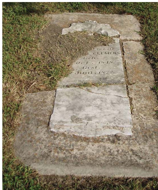
Figure 4-47. This headstone had broken off its base. Concrete slab into which it was laid has failed on the subsiding soil and caused further damage. JMA, 2009.
