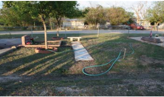
Figure 4-58. The presence of a hose attached to this hose bib indicates active use of the system. JMA, 2009.
