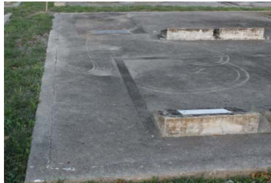
Figure 5-47. Concrete plot cover poured up to the curb level. Note wheel tracks left by a rider mower. JMA, 2009.
