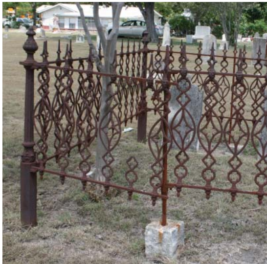
Figure 4-56. This cast iron fence has been damaged, possibly due to soil subsidence. JMA, 2009.
