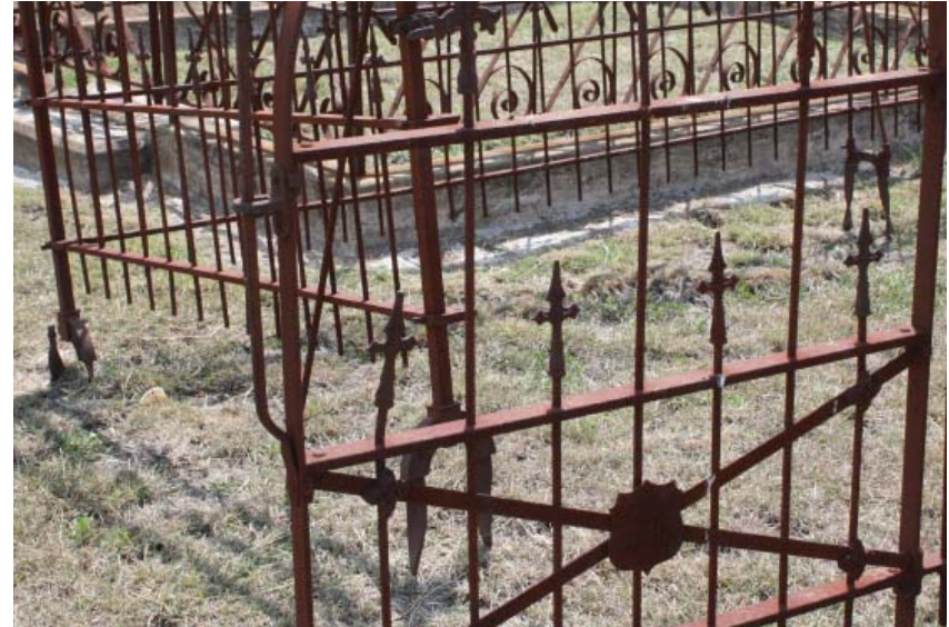
Figure 4-55. Soil movement has led to shifting and lifting of the anchoring system of this fence. JMA, 2009.
