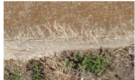
Figure 4-30. Metal-core string trimmer marks found in New Braunfels Cemetery JMA, 2009.
