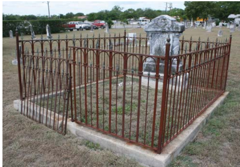
Figure 4-57. The gate of this fence has fallen off, but has been retained. JMA, 2009.
