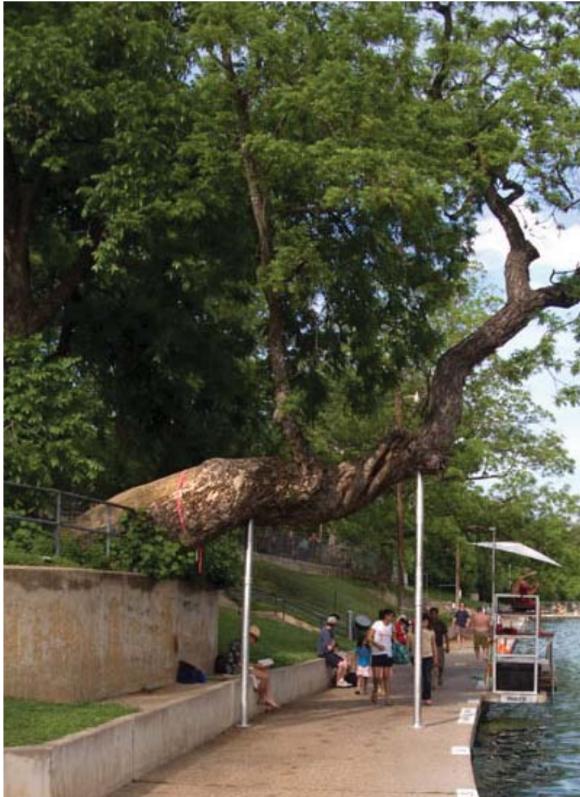
Figure 2-2. This pecan contributes to the historic character of Barton Springs in Austin and has been stabilized with steel posts. JMA Collection.
