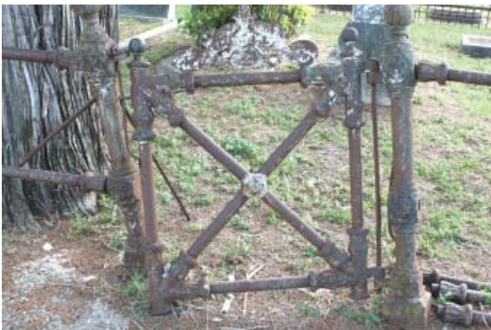
Figure 5-58. The gate in this unusual gas-pipe fence has been set askew due to shifting from vegetative growth. JMA, 2009.
