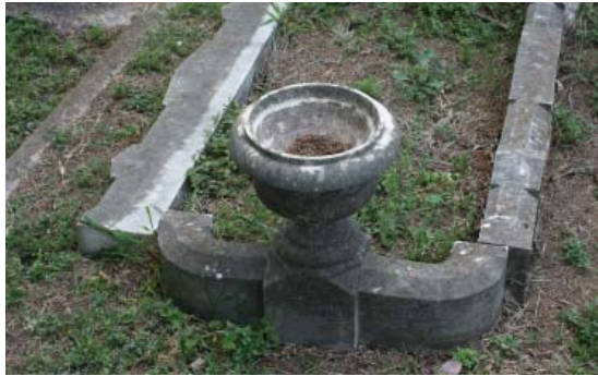
Figure 5-44. The pinning system for this marble curb has failed and the units displaced. JMA, 2009.
