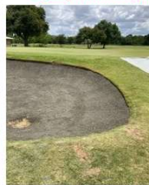
Capillary concrete is applied
