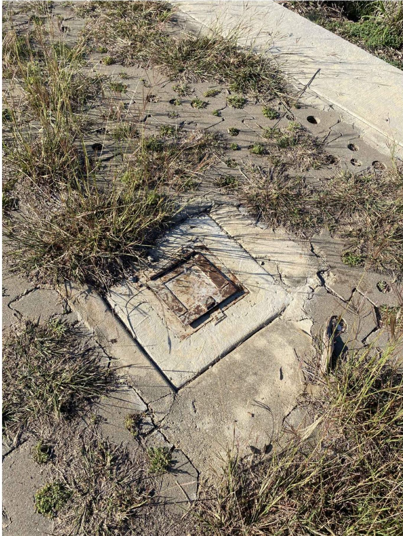
TYPICAL EMBANKMENT PIEZOMETER COVER CONDITION (PHOTO TAKEN ON APRIL 12, 2023)
