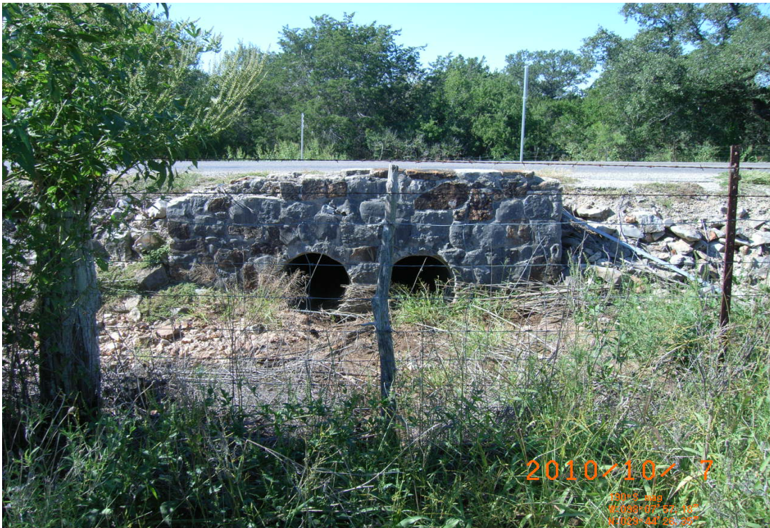
Culvert crossing at River Road.
