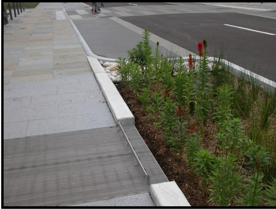
Figure 3-1 – Basic Rain Garden Components
